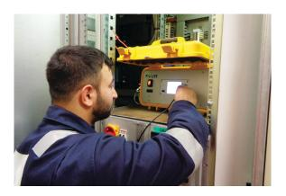
For older systems, Viper Innovations has designed a suite of 'Interface Modules' that allow the **V-LIM** to be easily integrated. These interface modules are fitted in place of the existing LIM and route the required electrical signals from inside the existing Power Module to front panel connectors.
